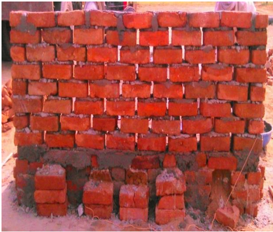
Fig 4: Outer wall of chamber
