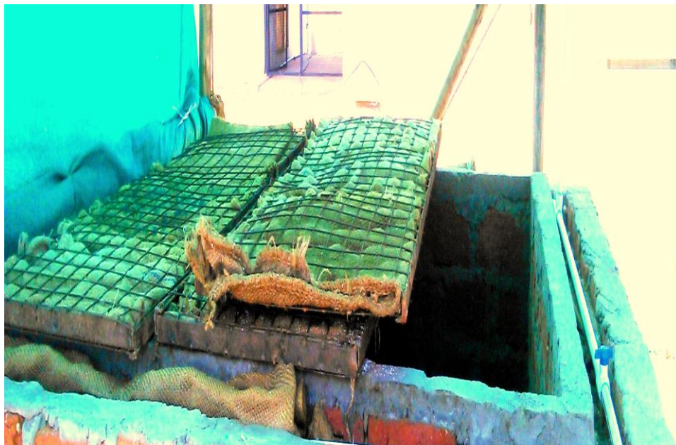
Fig 6: Gates are placed on cooling chamber
