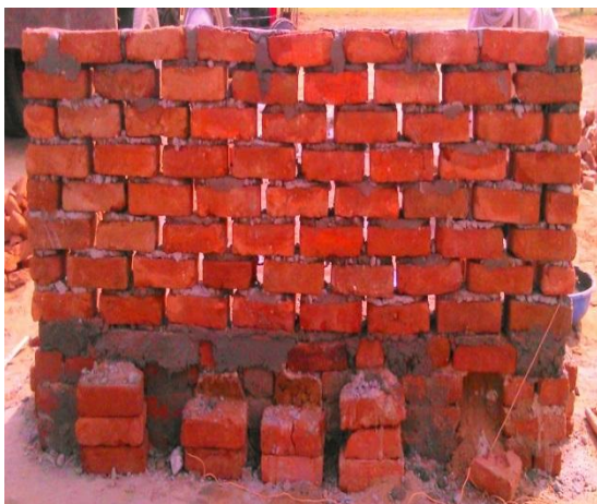
Fig 4: Outer wall of chamber
