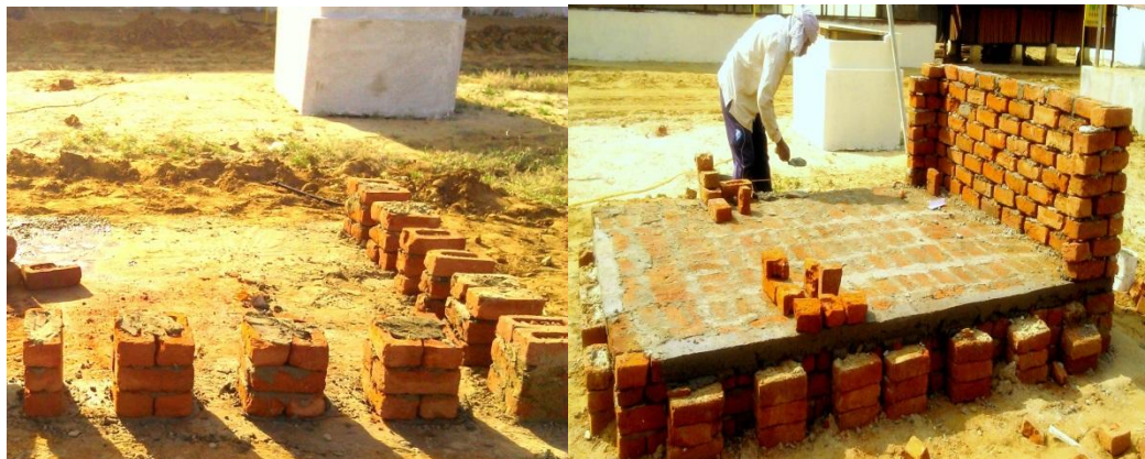
Fig 2: Main base with pillars
