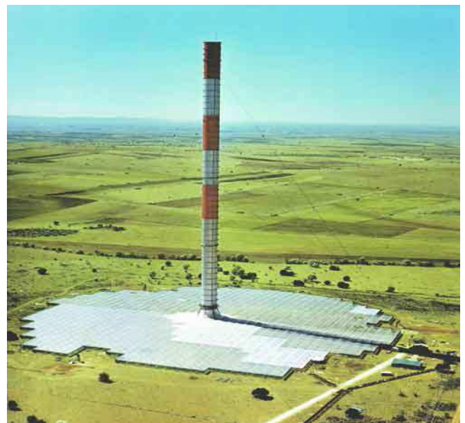
Fig.1. A view of the Manzanares Solar Chimney Power Plant
