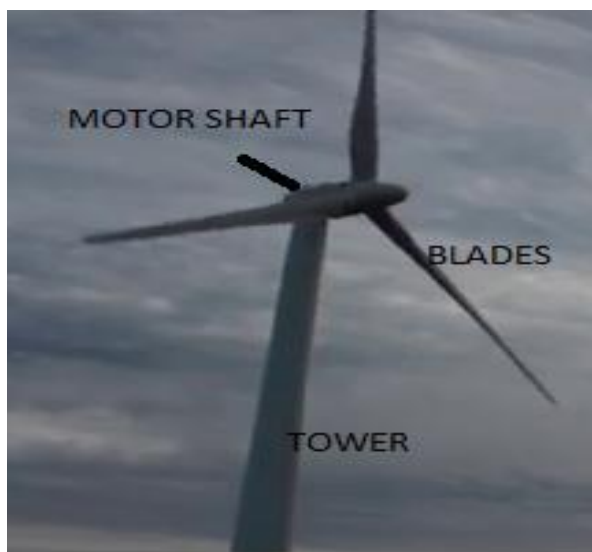
fig .1 wind turbine
