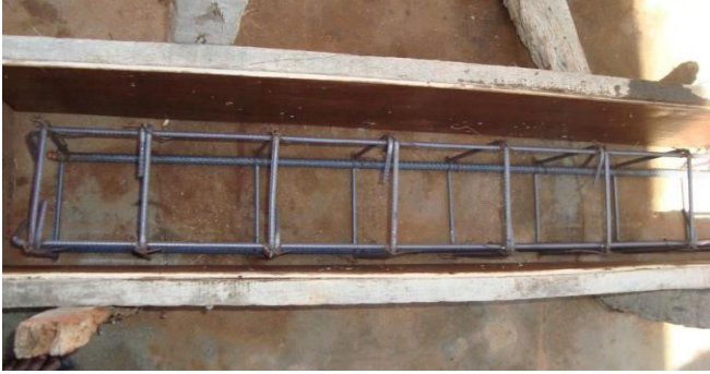
Fig 2 (a): Mould for Casting Specimen
