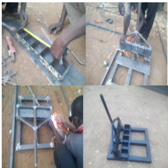
Plate 1: Moulder under and after construction processes.
